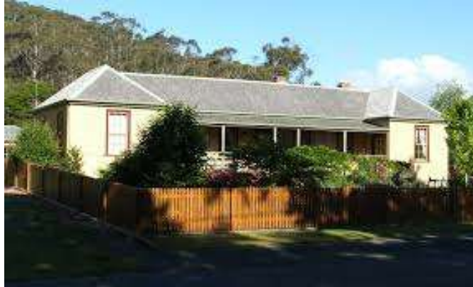
The relocated and renovated Sherwood Hall, Latrobe. Relocated by the Devon Historical Society.
